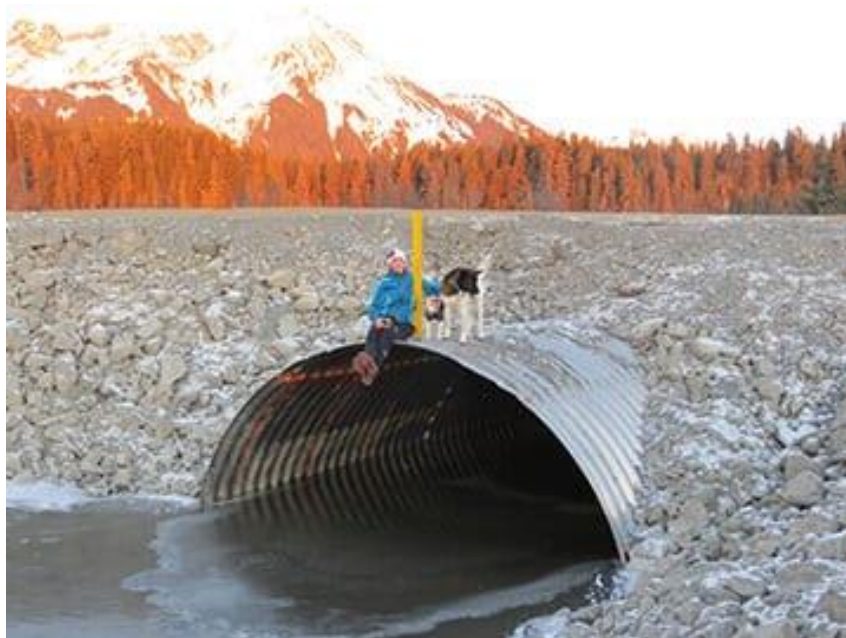
Fish-friendly culverts: Lined with streambed material, this culvert spans the full width of the natural stream channel, providing more natural conditions for fish passage. Photo: Copper River Watershed Project
